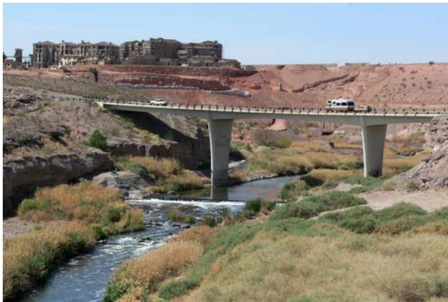
Northshore Road Bridge at the lower end of the Wash. (Wikipedia photo)
