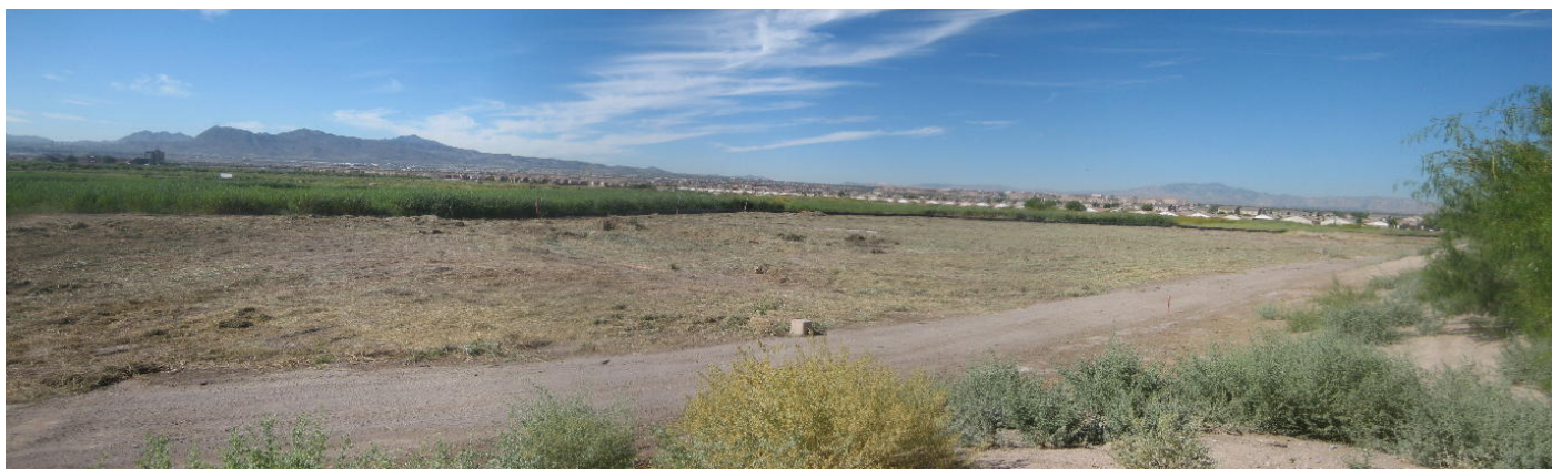
Panoramic view of the new Visitors Center construction site, just south of the east end of the Nature Preserve.
