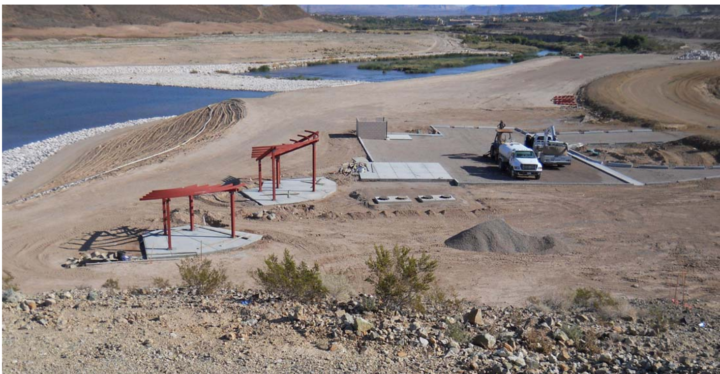
Wells Trailhead Construction (a Clark County Photo)
