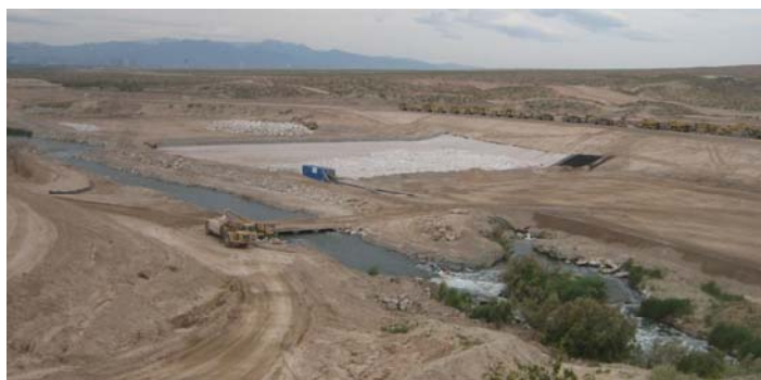
Lower Narrows Weir construction site
