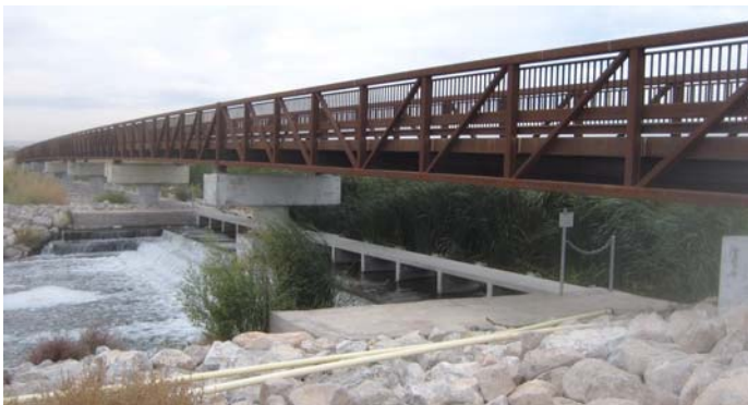
Upper Diversion Weir
