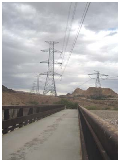
Powerline Crossing Weir Bridge
